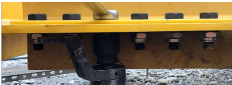
Installing ESL locknuts using hand tools
